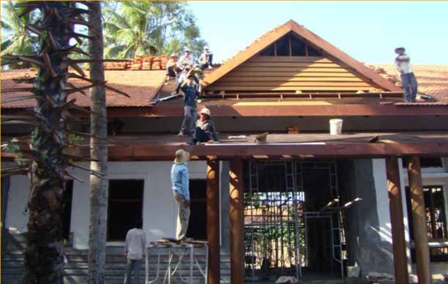
Putting on the roof before the rainy season
